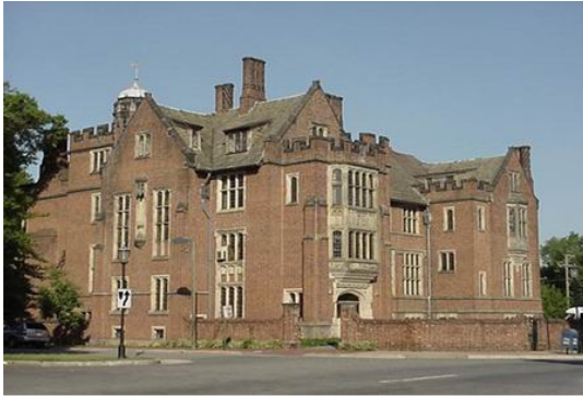
Branch House, Richmond VA
